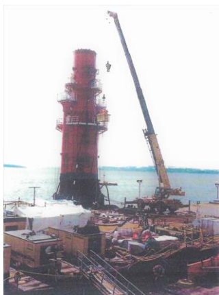
Ballasting of Fulmar loading bouy
